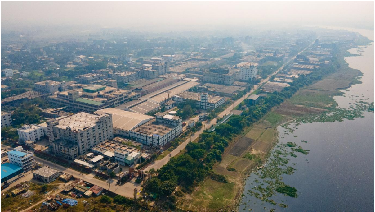
Photo 1: Aerial view of the Savar Tannery Estate
